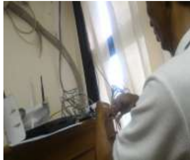
Gambar 3.2 Proses crimping kabel UTP
