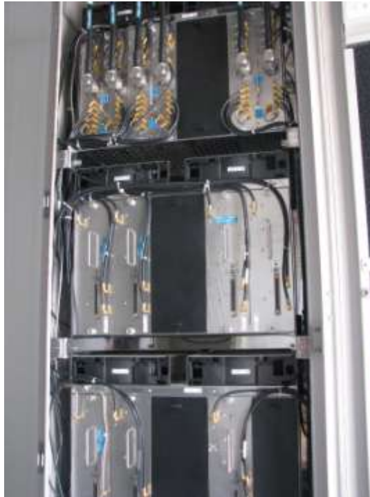
Gambar 3.7 Base Transceiver Station (ekoyw, 2011)
