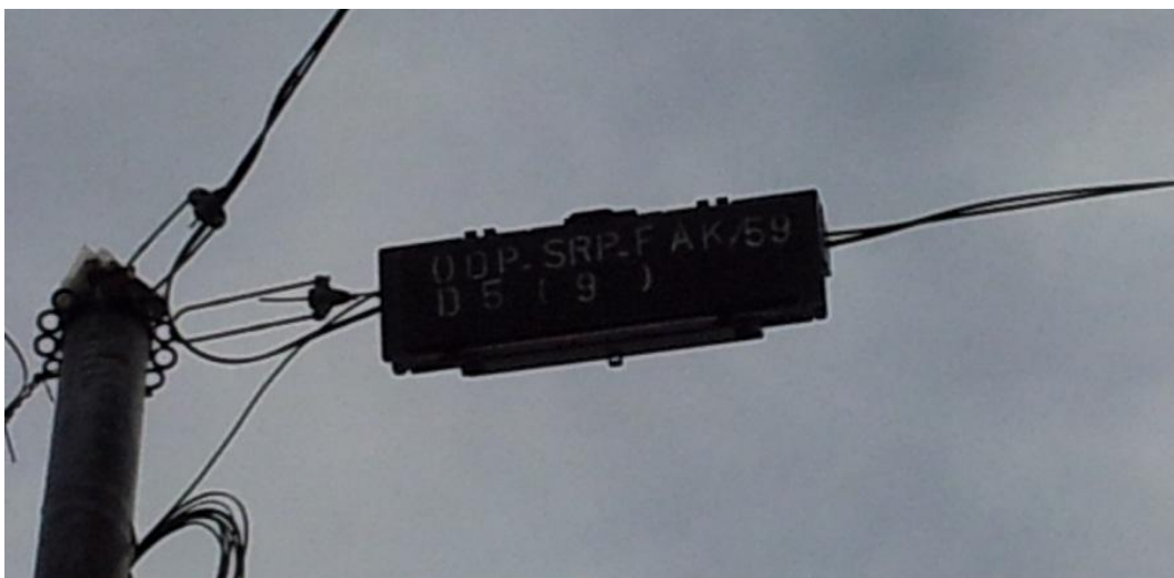
Gambar 3.2 Optical Distribution Point (ODP)
