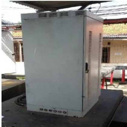
Gambar 4.3 Perangkat Box RBS outdoor
