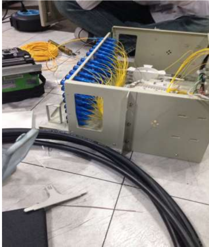
Gambar 3.5 Penginstalan Tieline
