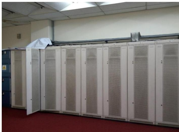
**Gambar 3. 2 LIM (Line Interface Module) dan GS (Group Switch)**
