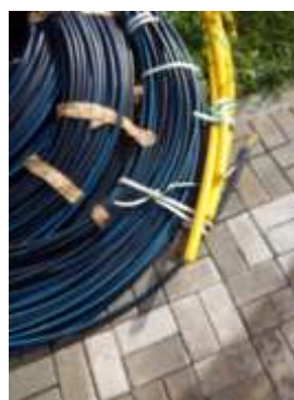
Gambar 3.5 kabel duct dan subduct
